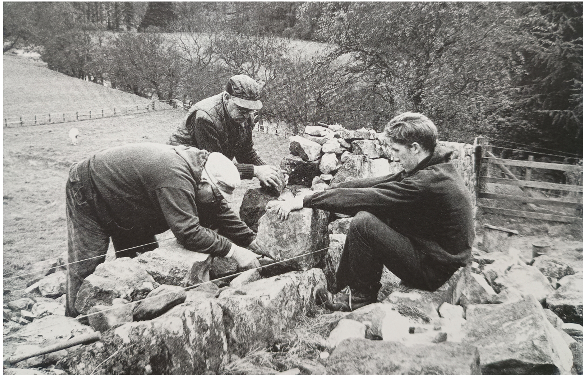
Three generations of Wallers: George, Thomas and Tom Hall of Coquetdale in mid-Northumberland. Halfway along a drystone wall at Park Hall Farm
